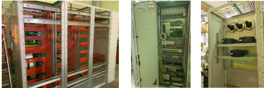
Figure 5: Enclosure (left) and LV (central) and HV (right) Modules in Progress
