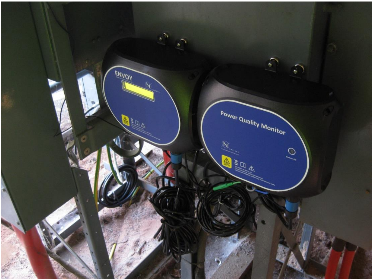
Figure 2-4: Plug & play PQ monitor installation at an 11 kV distribution substation
