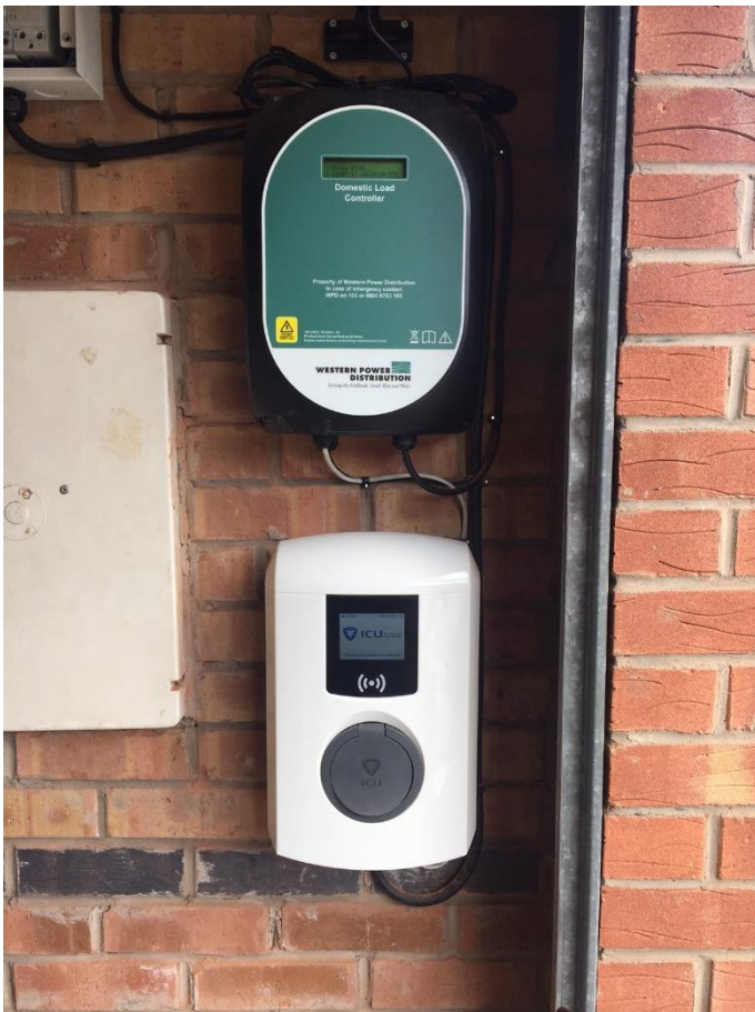
Figure 2-1: Example Installation of Project Equipment: A Controllable EV Charge Point and Domestic Load Controller
