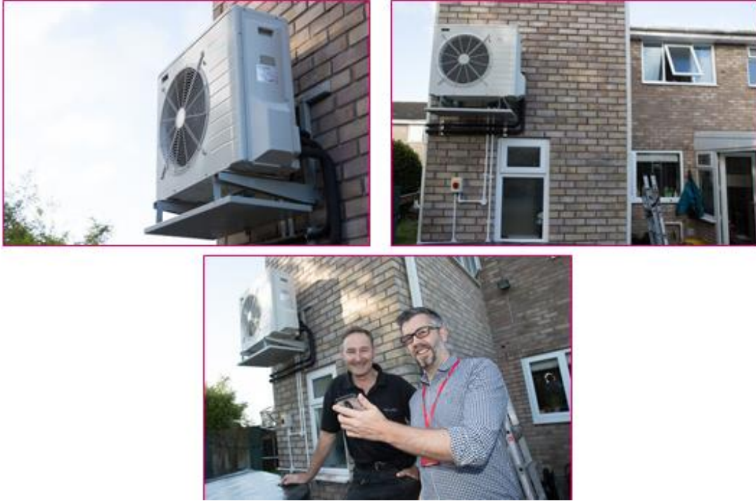
Figure 2: Daikin units installation
