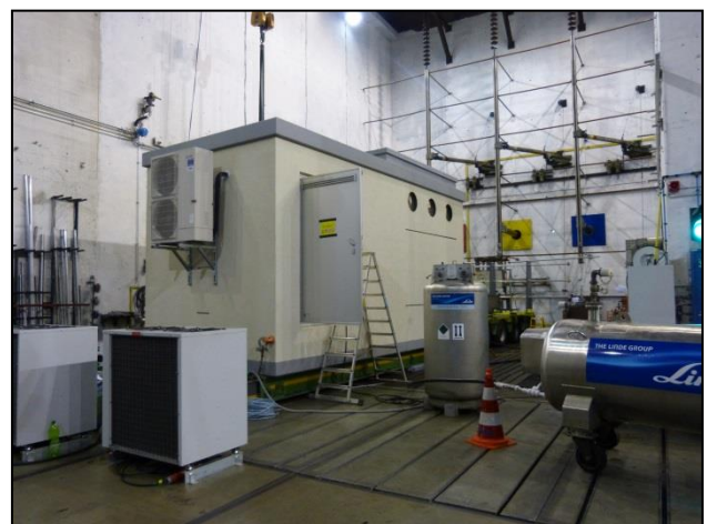
Figure 2: RSFCL during short circuit testing at the KEMA laboratory, Arnhem, Netherlands
