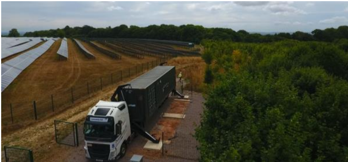
Image 14 - Battery lift and loading on to transporter
