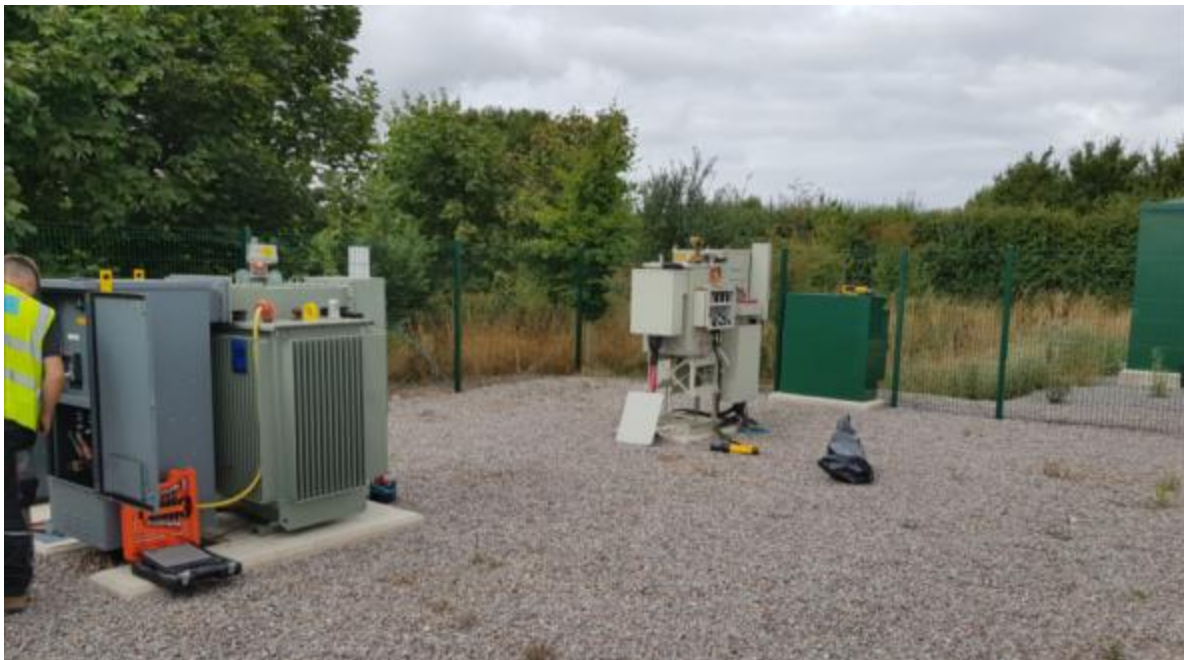
Image 9 – Day 1, BSR Engineers isolating and disconnecting ancillary assets
