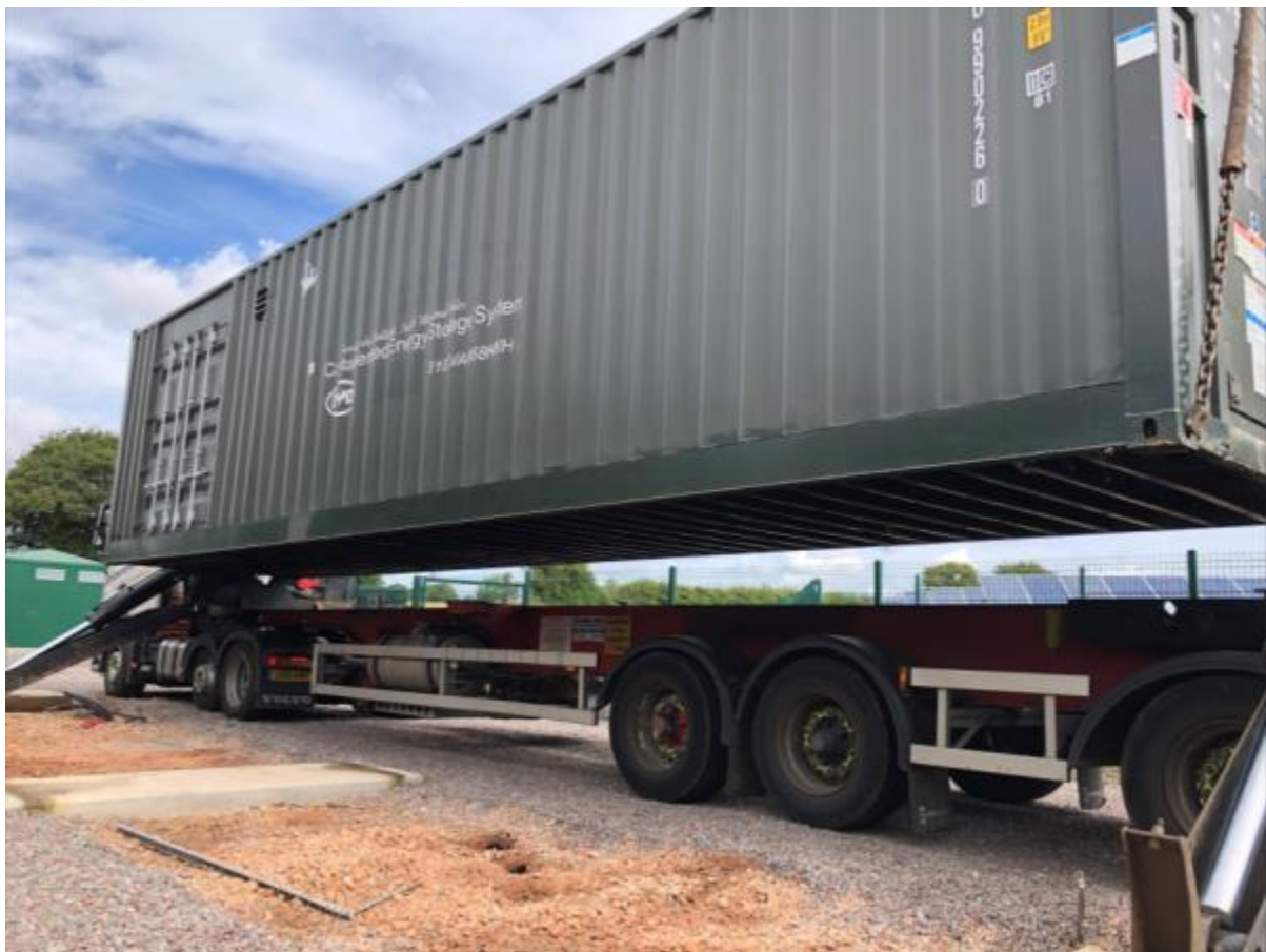
Image 13 - Ground level view of lift in progress
