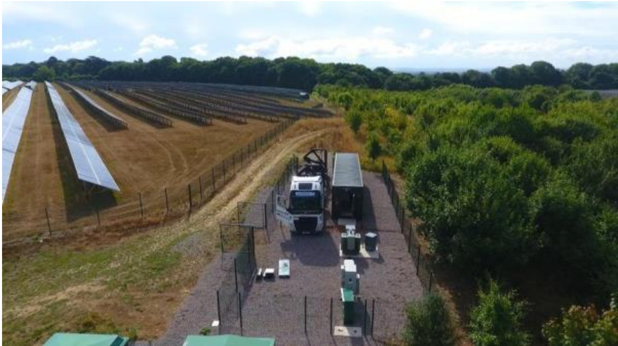
Image 12 – Aerial view of vehicle aligning with battery and setting outriggers
