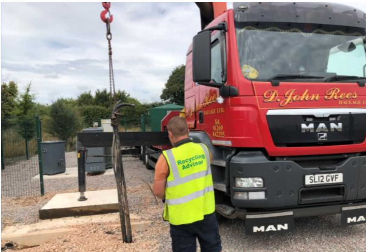
Image 17 - Removal of cable tails from ducting
