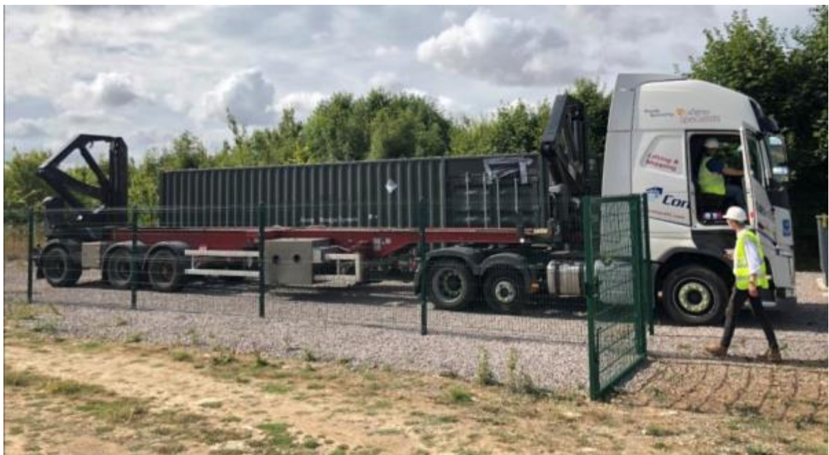
Image 11 – Uplift vehicle aligning with battery and setting outriggers
