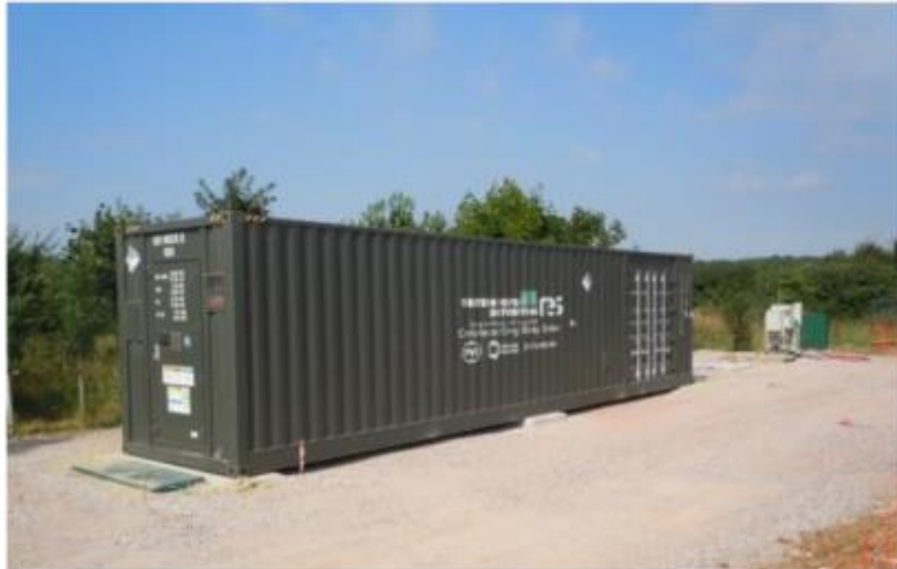
Image 4 - Plinth mounting prior to Fencing install
