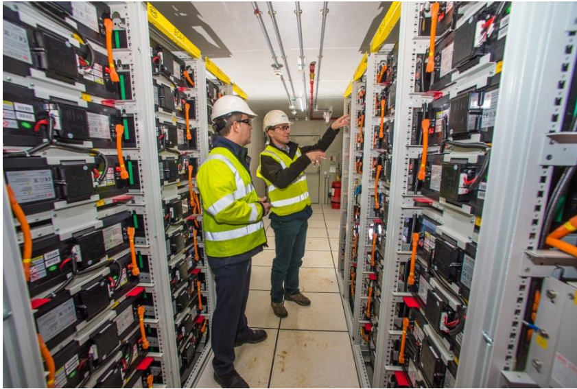
Battery strings and fire suppression system.
