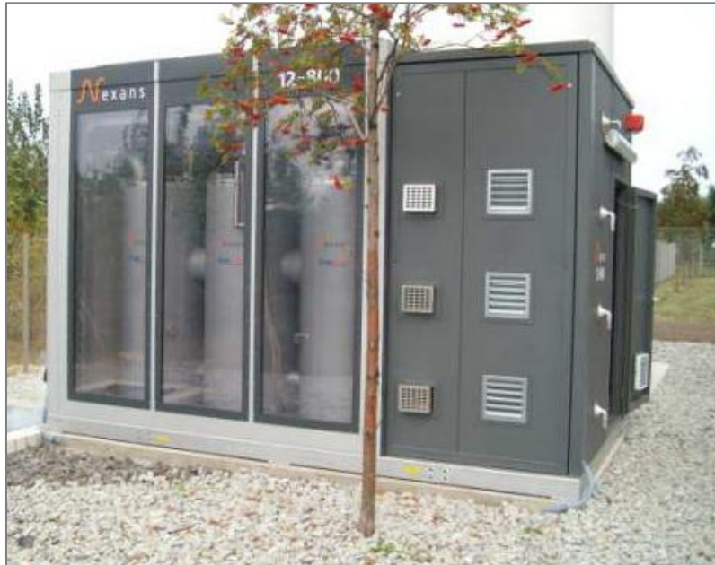
Figure 3-2: Example of a RSFCL
