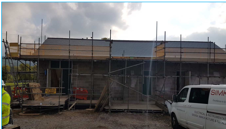
Figure 2-19: Construction of 33kV switchroom in early May 2017
