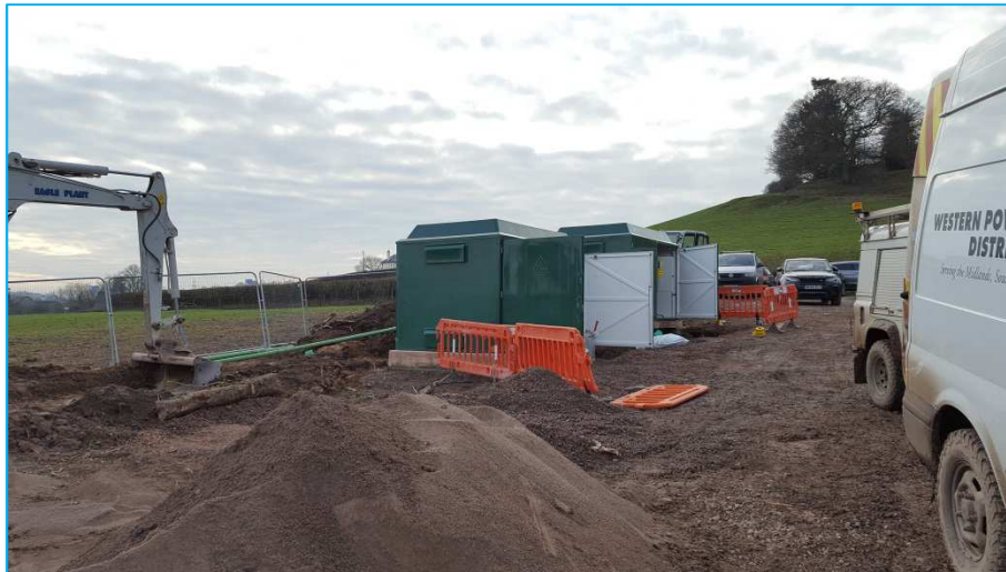
Figure 2-18: Installation of Distribution Substations during February 2017
