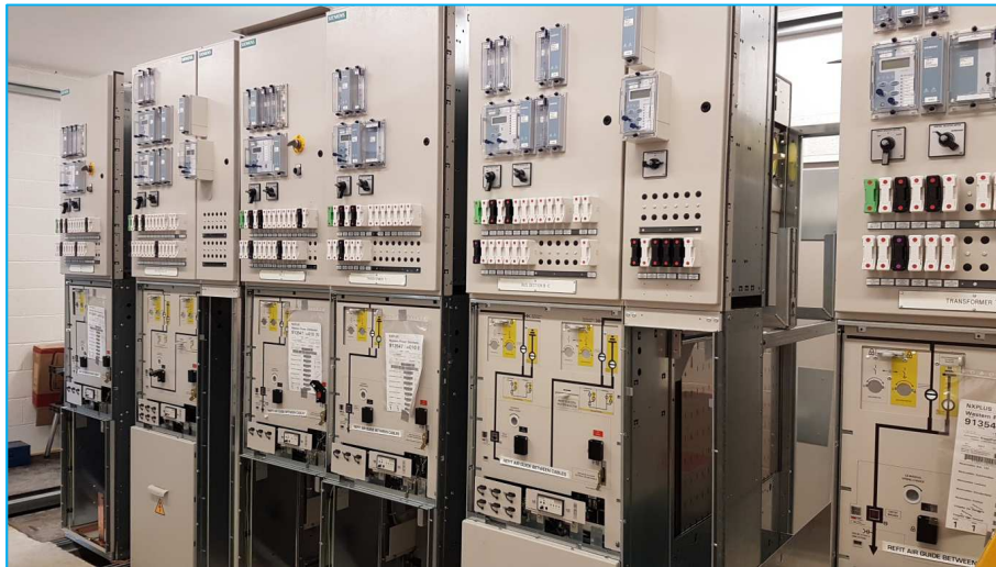
Figure 2-20: 33kV switchgear being installed at Exebridge
