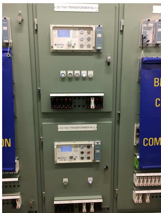
Figure 2-6: Picture of combined T1 and T2 AVC Panel with SuperTAPP SG Installed
