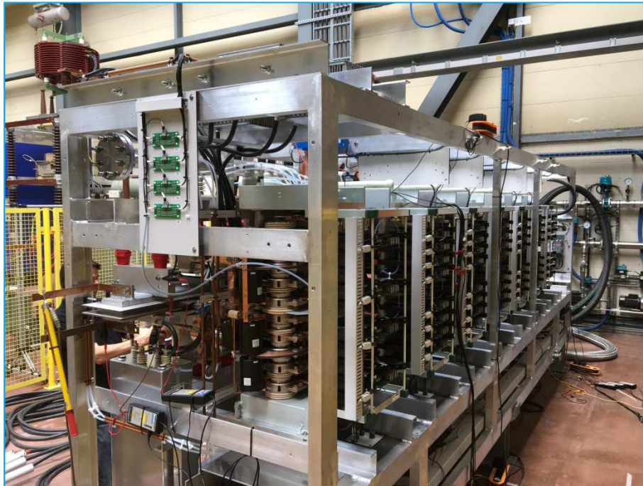
Figure 2-16: Converter Frame prepared for testing
