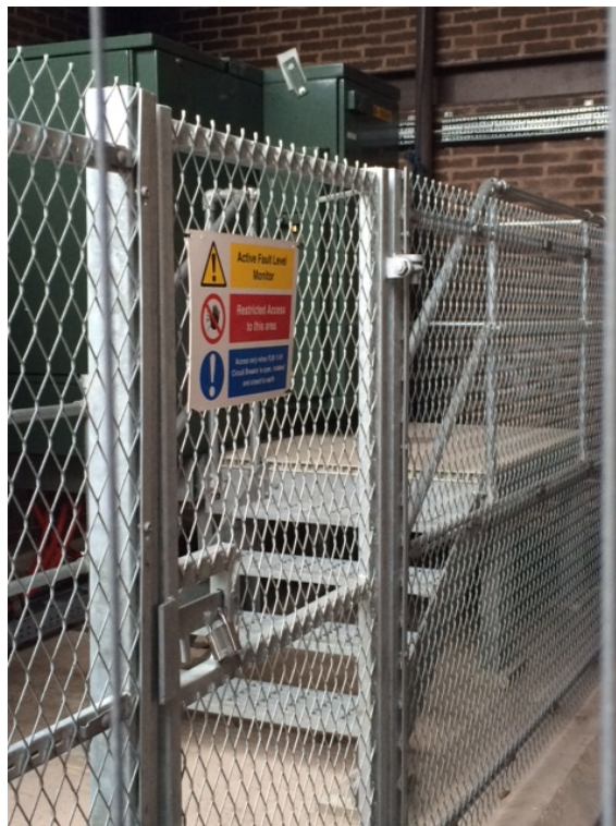
Figure 6-4 - FLM 11kV Compound Access
