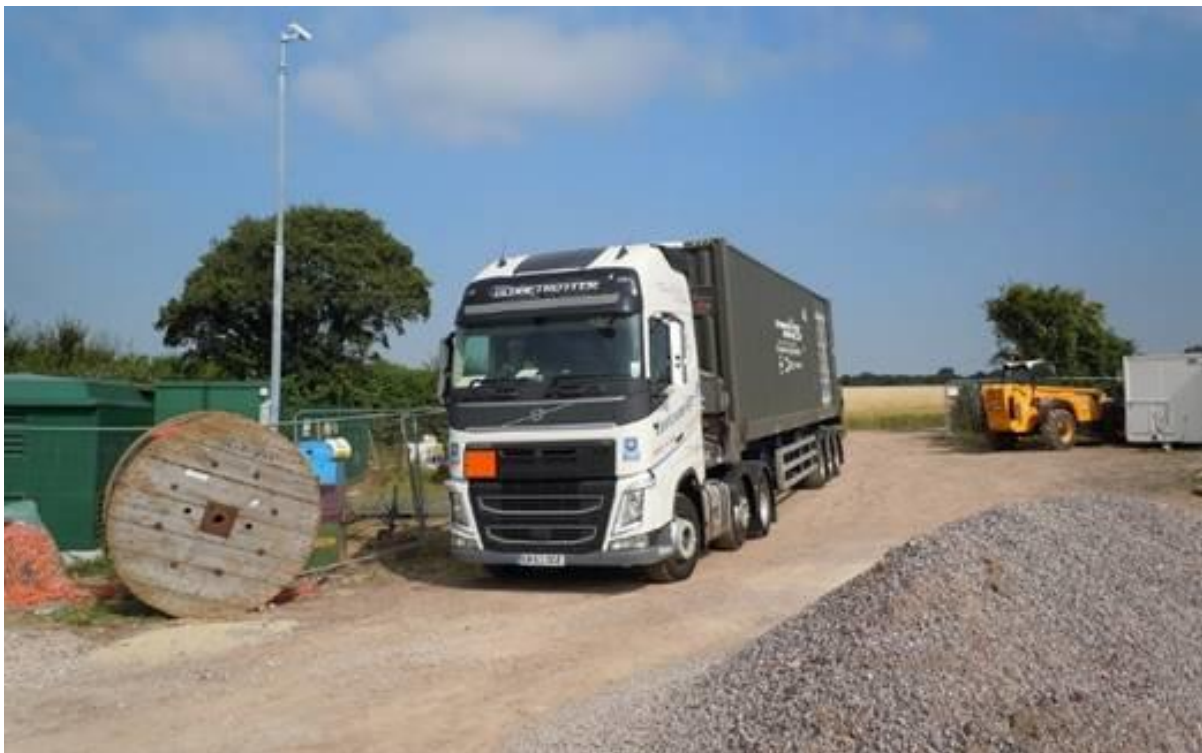
The photograph shows some key stages of the construction
