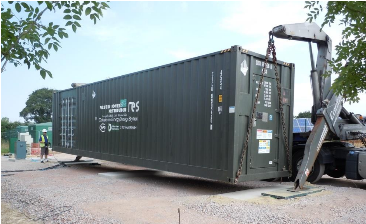
Battery arrival and offloading
