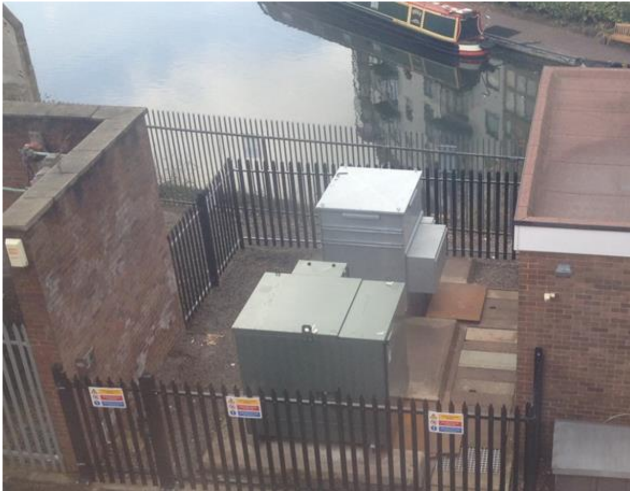
Ladywood FLM Installation
