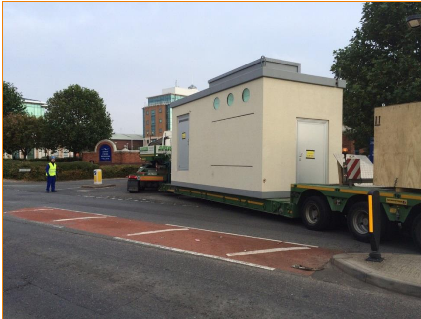
Figure 8-1: Chester Street FCL being delivered to site
