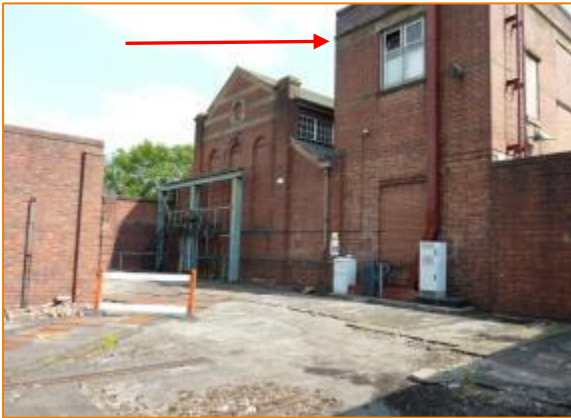
Figure 5-11: Substation building as seen from the disused transformer yard (first floor switchroom indicated by red arrow)
