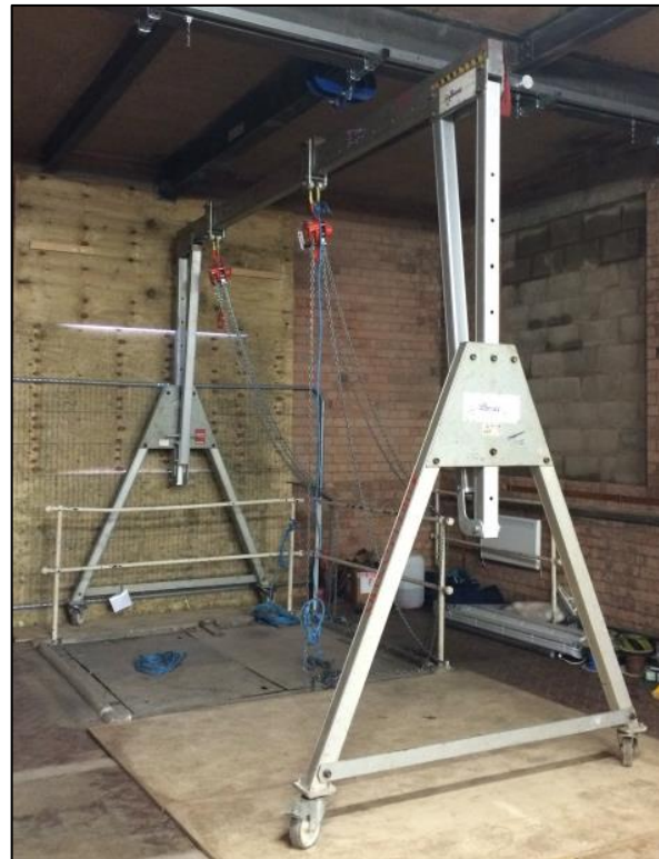
Figure 7-8 – Portable lifting frame used to lift the cryostat vessels to the first floor
