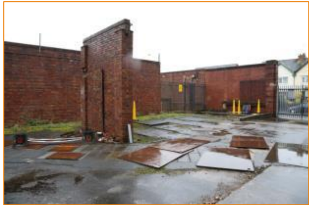
Figure 5-12: Disused transformer yard
