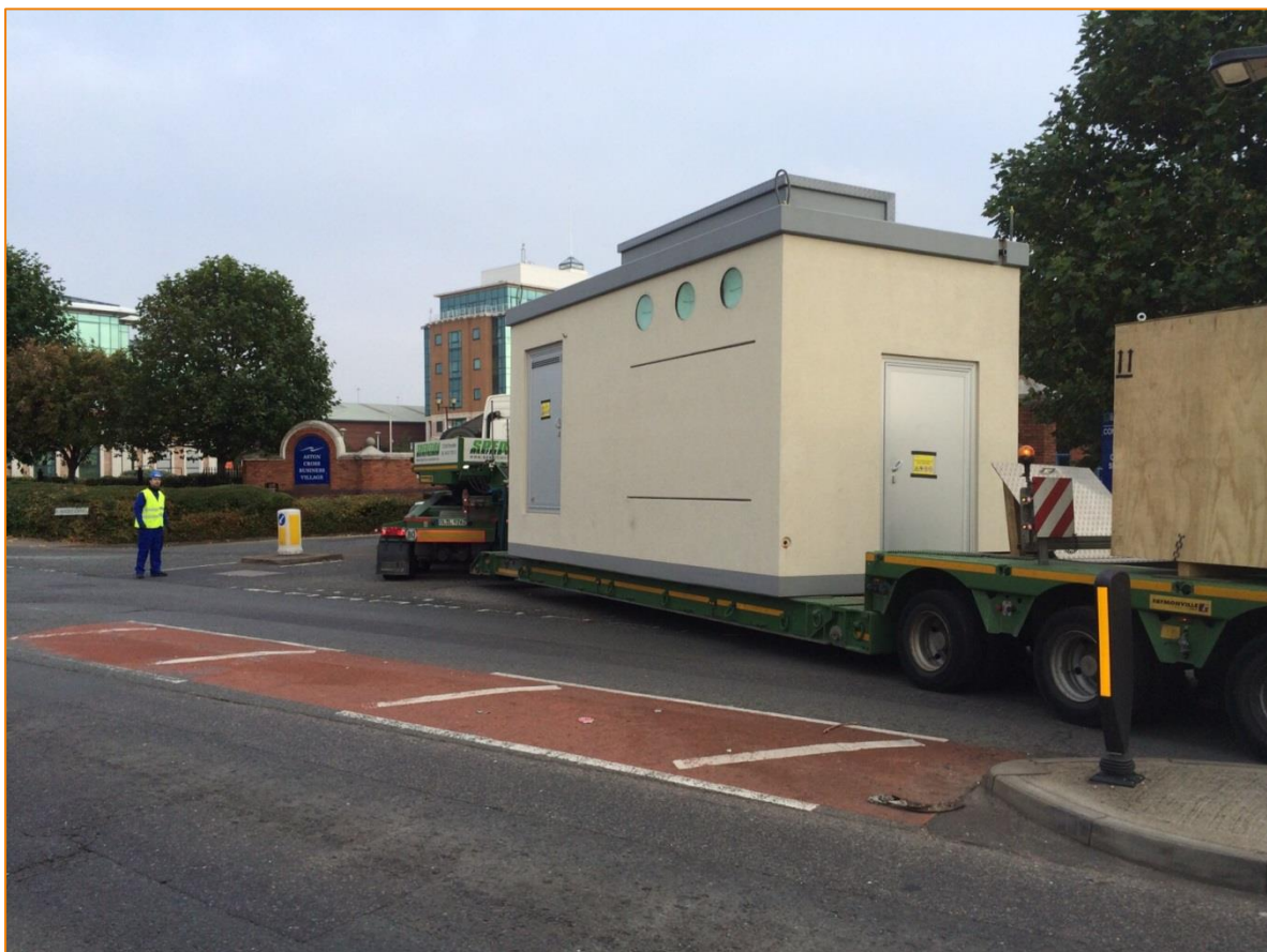
Figure 7-4: Chester Street FCL being delivered to site
