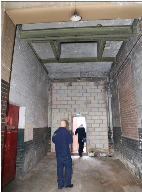
Figure 7-7 – Area underneath first floor equipment lifting hatch
