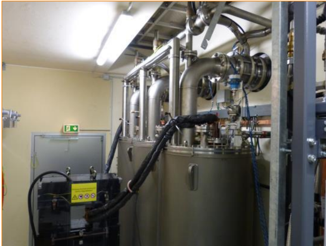
Figure 6-4: RSFCL undergoing current testing at the Nexans factory in Hanover
