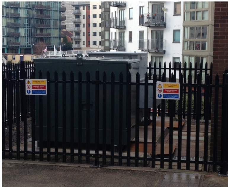
Figure 4-10: AFLM Installation at Ladywood – Side View
