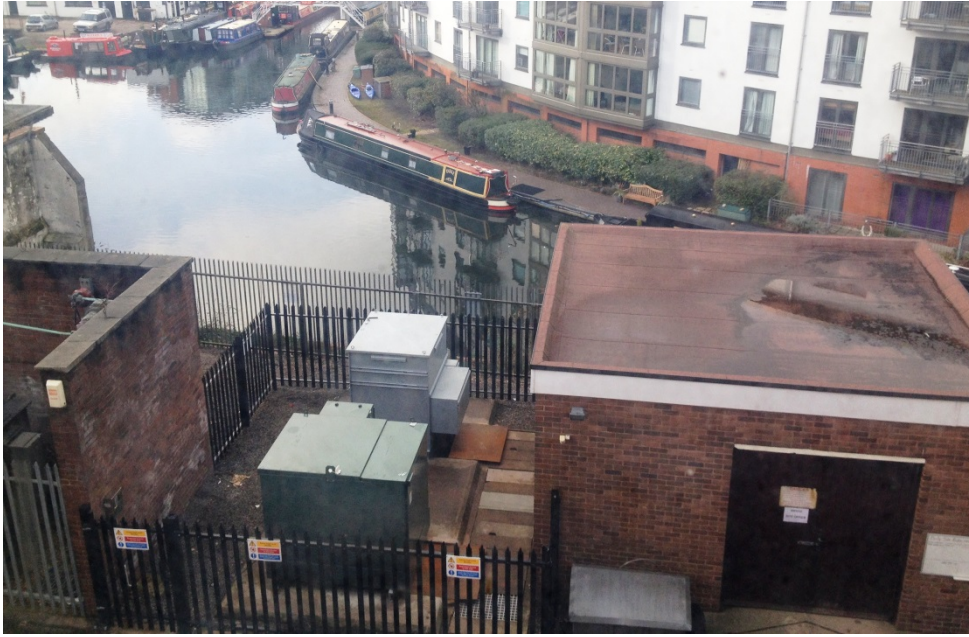
Figure 4-11: AFLM Installation at Ladywood – Top View
