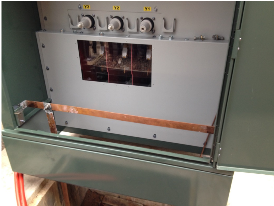
Figure 4-12: Earth bar upgrade of Pad-Mounted Style IntelliRupter® PulseCloser
