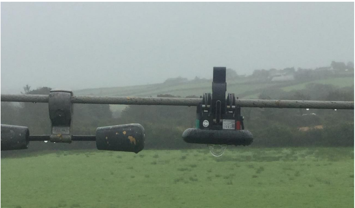
Figure 2-2 – HV SN2.0 installation on 132kV circuit - 175mm 2 ACSR conductor
