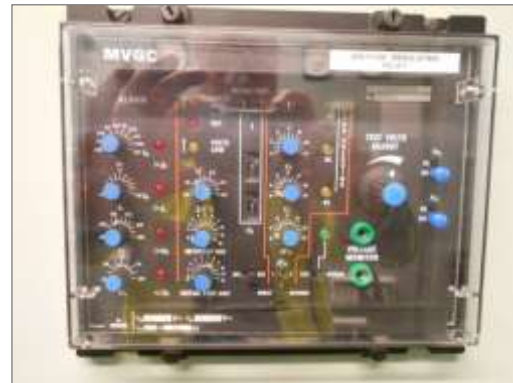
Figure 5-2: MVGC01 AVC Relay
