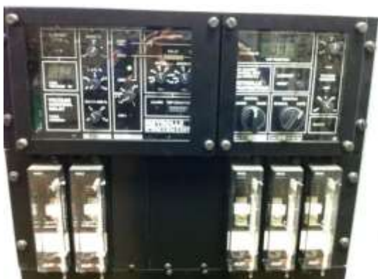
Figure 5-5: Reyrolle SuperTAPP AVC Relay
