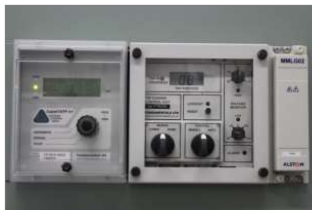
Figure 5-6: SuperTAPP n+ AVC Relay
