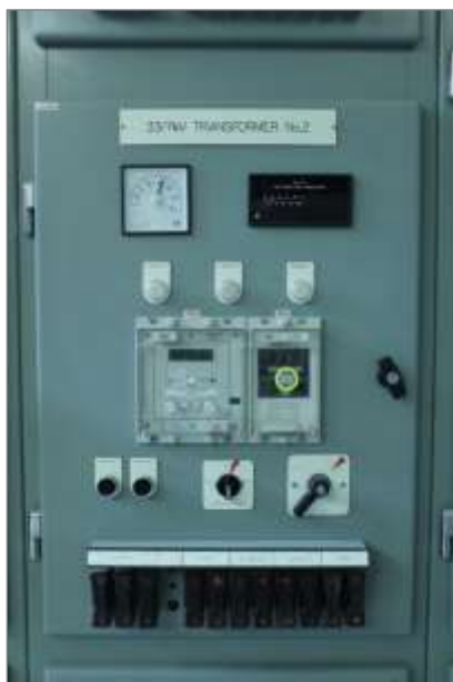
Figure 5-3: KVGC202 AVC Relay
