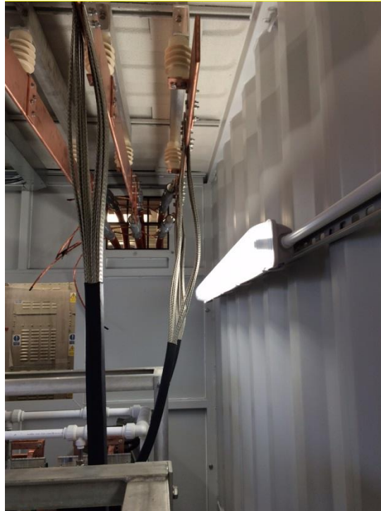
Figure 2-21 - Alstom AFD 11kV Braiding
