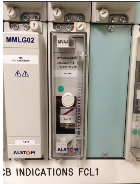
Figure 2-16: Trip Relay Operation
