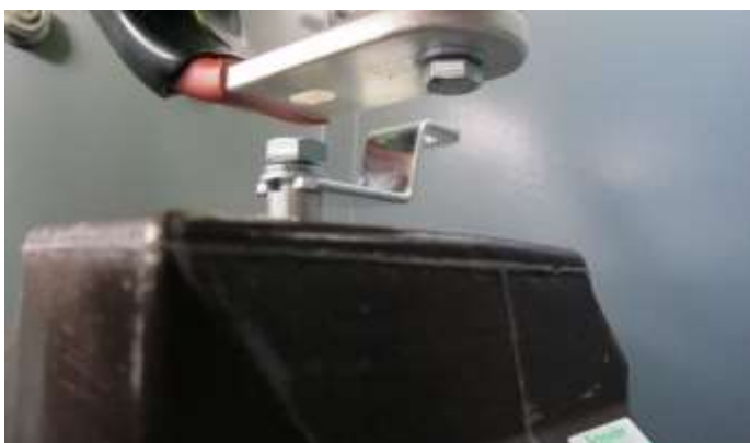
Figure 7 : RMU VT compartment.
