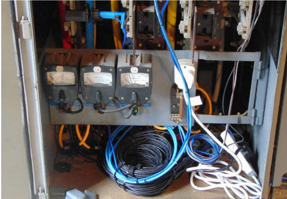
Figure 18: Securing excess cables in the LV cabinet at Pilgrim Drive substation
