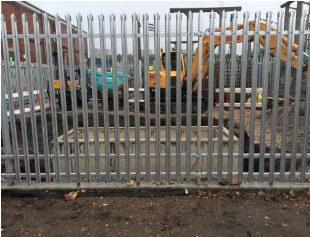
Figure 2-14 - FCL and FLM area with new palisade fencing
