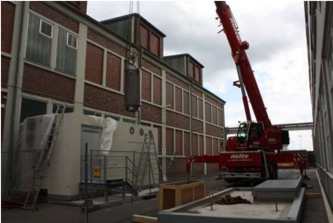
Figure 2-10 - Cryostat being installed in the FCL enclosure
