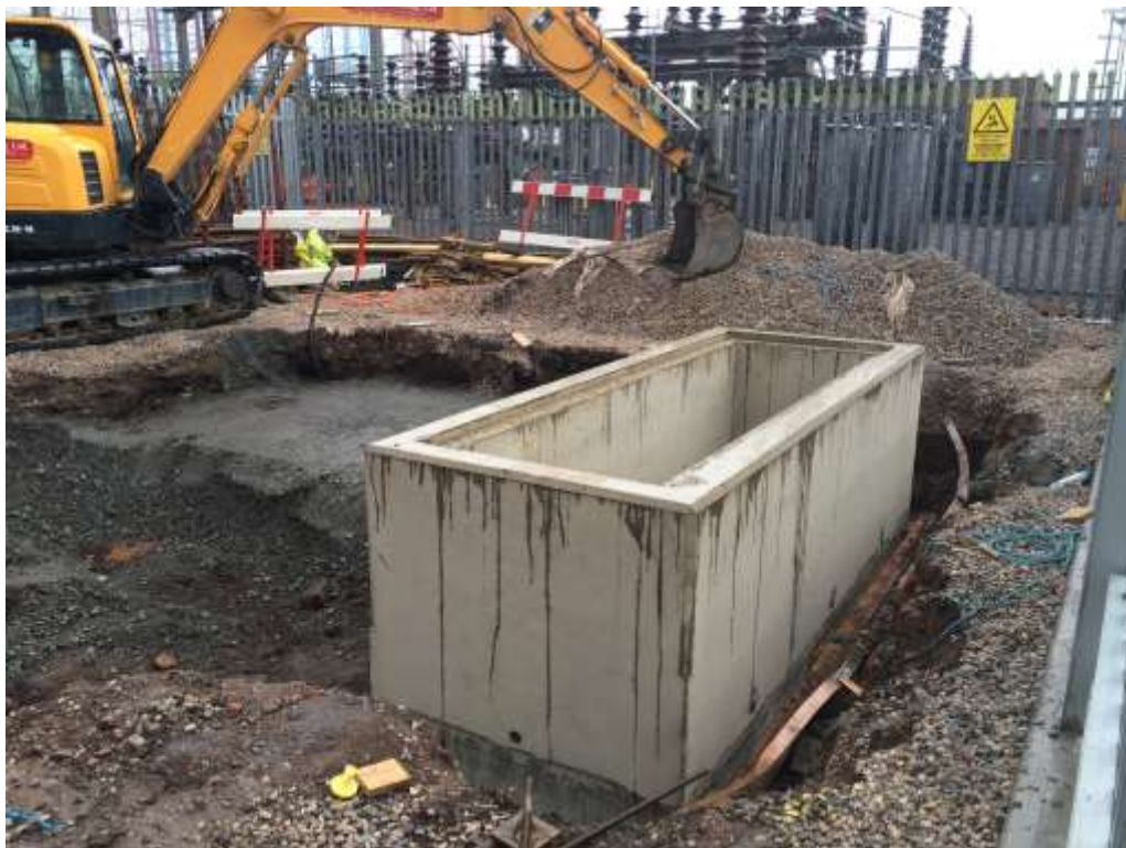
Figure 2-15 - Concrete casting of FCL pressure relief bund
