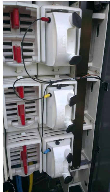
Figure 18: Modified Fuse Carrier
