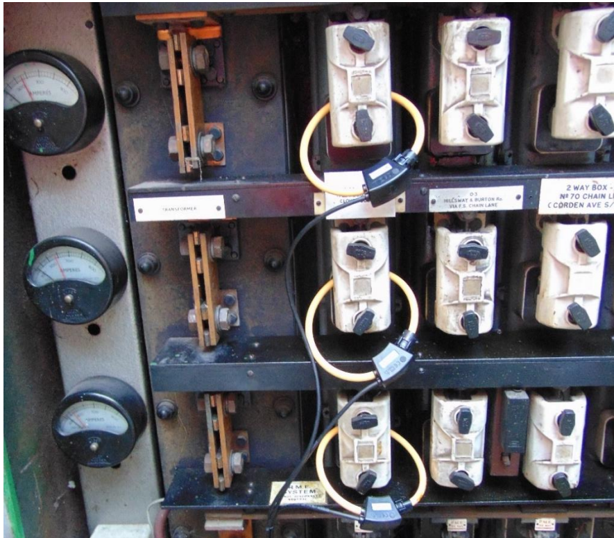
Figure 22: Flexible Rogowski Coils installed around fuse carriers
