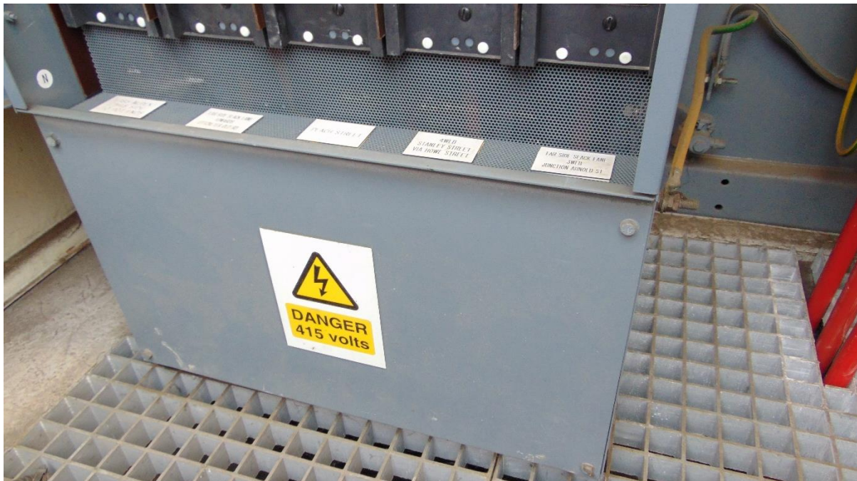
Figure 14: LV Enclosure Panel
