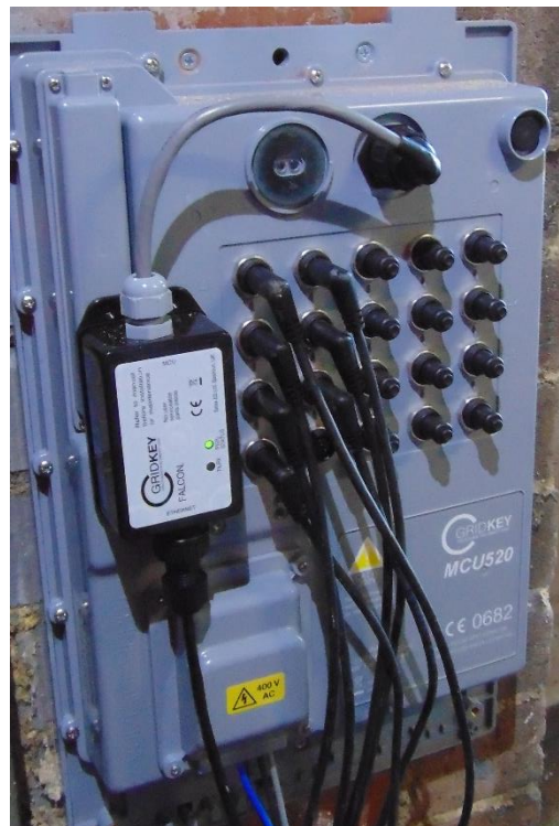
Figure 25: GridKey MCU520 Connections
