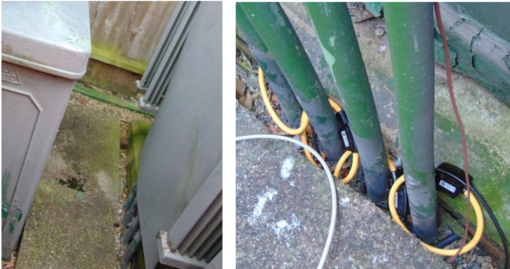
Figure 23: Transformer – LV Board Monitoring
