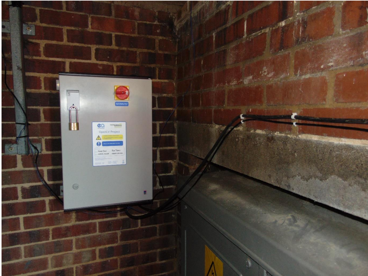
Figure 10: Example of wall-mounted enclosure
