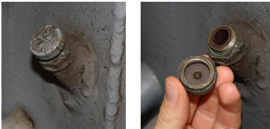
Figure 7: Example of a transformer oil pocket and cap
