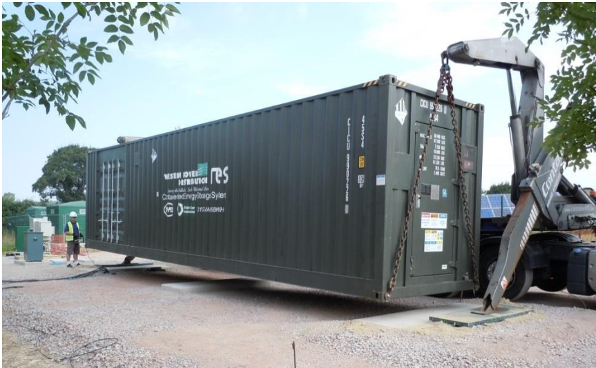
Figure 6: Battery Offloading
