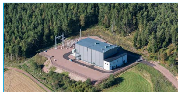
Figure 5-10 – Åland converter station
