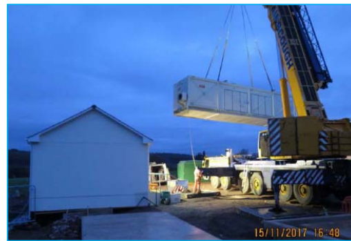
Figure 7-5 – delivery of the FPL container
