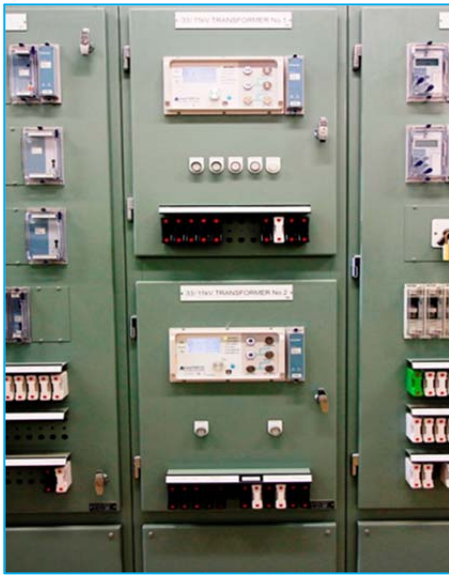
Figure 6-5 – SuperTAPP SG relay installation
