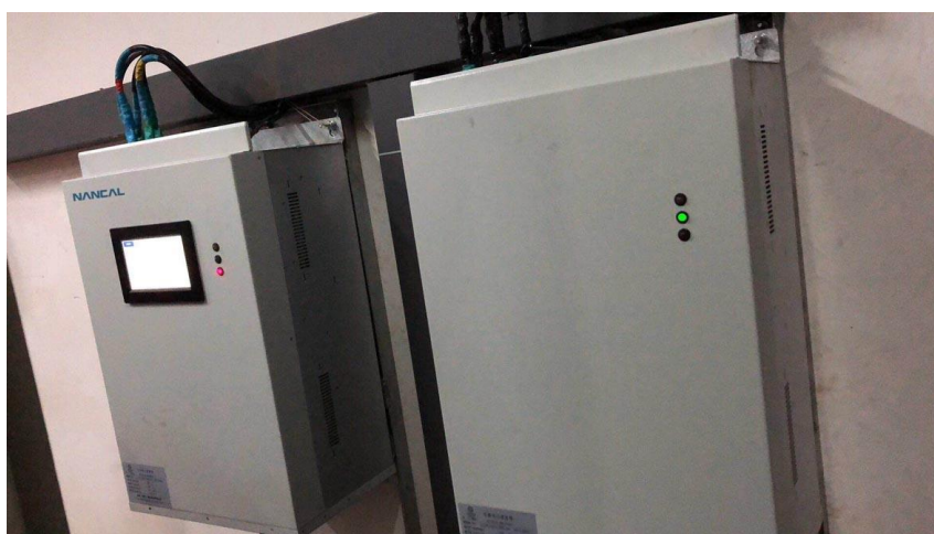
Figure 36: Wall mounted low power AF used in hospital manufactured by NANCAL [106].
