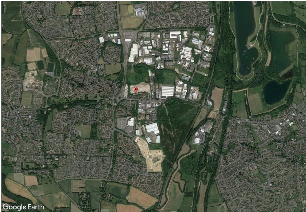
Figure A 7: Halfway 33 11 kV S Stn
