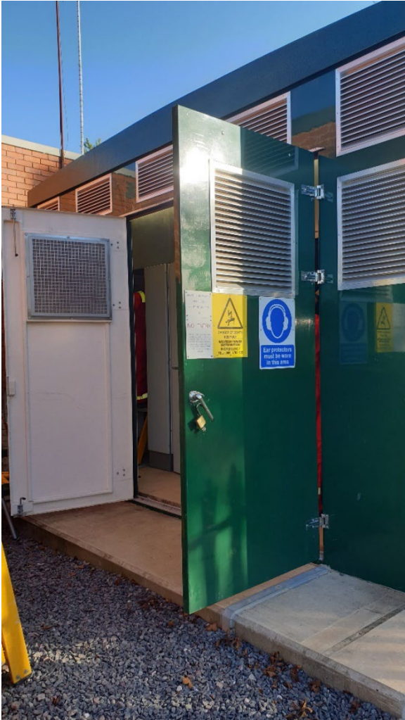
Figure 2-3 Image showing EDGE-FCLi during remedial work site visit
