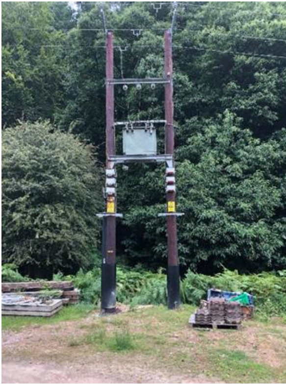
Figure 13 Image of Pole Boar Guard Installations in the Forrest of Dean
