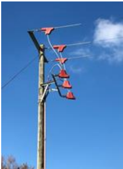
Figure 15 Photograph of the completed trial installation
