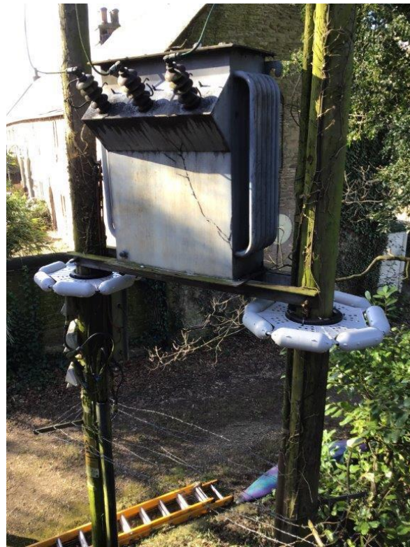
Figure 14 Carnfield Hall Poleguard installation
