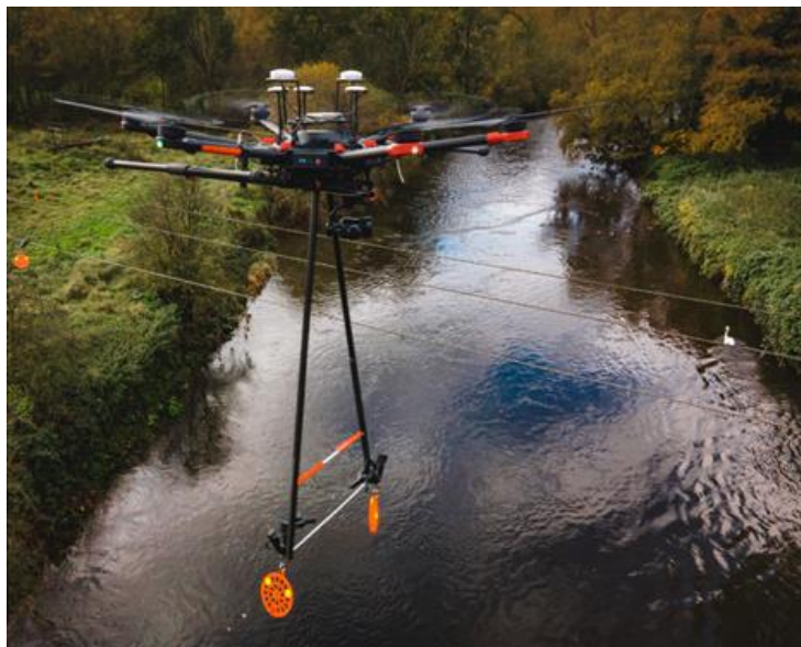
Figure 11 Drone installation of the Crocfast Bird Flight Diverters
