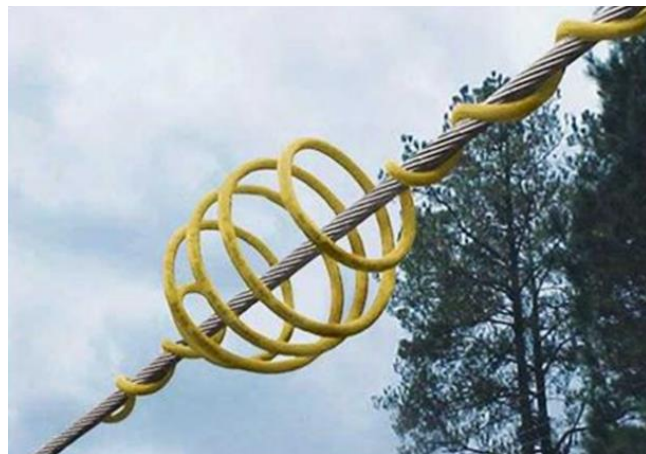
Figure 5 an example of a swan flight diverter
