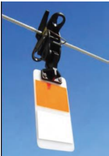
Figure 6 an example of a static bird flight diverter
