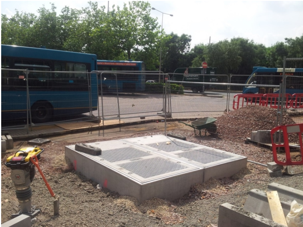
Fig 6 : Bletchley Installation Progress
