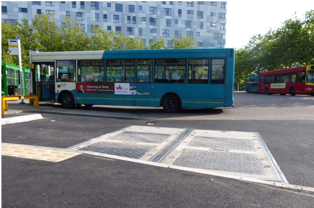
Fig7: Bletchley Station Final IPT installation
