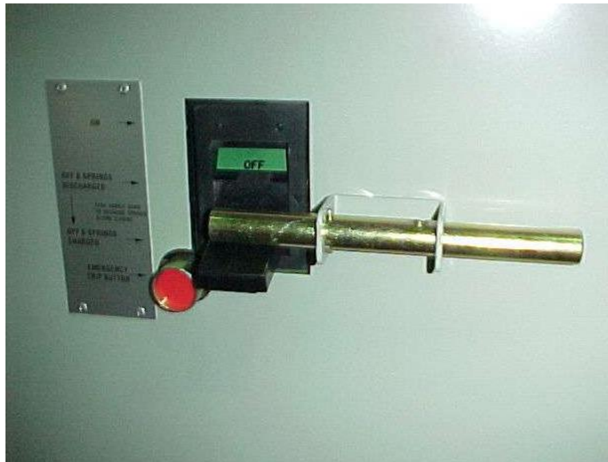
Figure B2 Metering MCCB Locking Arrangement
