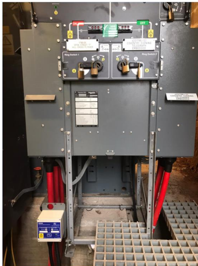
Figure 6: Example of NX44 installation
