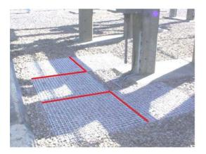
• Bolt the individual gratings together using five stainless steel fixings per side. The fixing arrangement shall be as per the following sketch.
