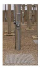
An operator stands in a fairly stationary position whilst operating the switchgear and consequently a single 1m x 1m grating shall be provided. The grating shall be aligned centrally relative to the sweep of the operating handle, with the closest edge located 500mm horizontally from the fulcrum.
