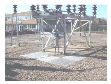
An operator "walks around" whilst operating the switchgear and consequently five 1m x 1m gratings connected together to form a "C" shape shall be provided. The gratings shall follow the sweep of the operating handle, with the closest edges located 500mm horizontally from the fulcrum.
