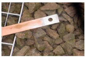
• Apply contact grease to the end of the earth tape and bolt to the grating
