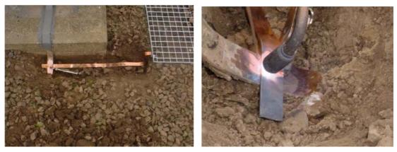
• The electrical connection should be readily visible for inspection. If the connection is likely to present a tripping hazard then it should be lightly covered with chippings in order to reduce the risk. The chippings should be able to be easily removed by hand so that an operative can verify the presence of the connection prior to carrying out a switching operation. If the electrical connection is not covered by chippings, then it should be painted grey to deter theft.
