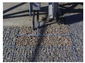
• Braze to the earth tape going direct to the switch handle mechanism. The brazing should be in accordance with the requirements of Standard Technique ST: TP21L Fixed Earthing Systems - Construction Techniques – Jointing.
