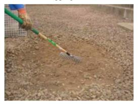
• Create a level base 30mm below the finished level of the chippings either by reinstating some of the removed chippings or by excavating some of the subsoil (as appropriate, depending upon the depth of the chipping layer). Place the grating in position, checking that it is 500mm (±50mm) horizontally from the handle fulcrum position and that it is level in all directions. Check that there is no inadvertent contact between the grating and any other earthed metalwork.
