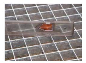
Reinstate the chippings around the side of the grating in order to hold it in position. The grating should, so far as is reasonably practicable, be "flush-fit" with the surface of the chippings so that it does not present a tripping hazard.
