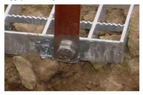
• Two connections are required on "C" shaped gratings, one at each end
