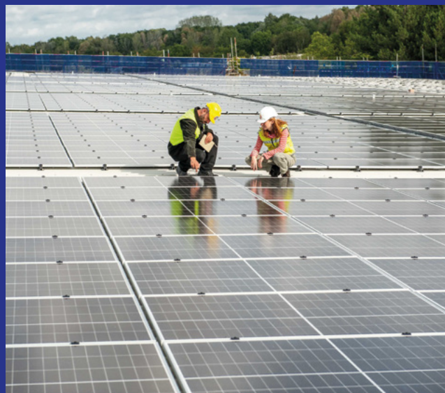
Image source: The Bottle Yard roof. Bristol Energy Cooperative.
